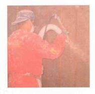
By blowing the insulation into sidewalls and other cavities, the insulation fills the cavity completely, eliminating voids frequently occurring with longer fibered materials. The short fibers flow freely around wires, switch boxes, rough plaster, and nails. In addition, Mountain Fiber Cellulose Insulation may be blown at a greater than settled density. This full density remains constant throughout years of service.
